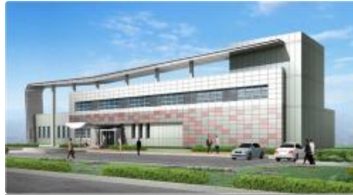
GIDC, Mongolia (2009) - Construction
